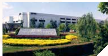
■ 北京第三工厂/The third factory 占地面积/Total land area: 274,579m 2 建筑面积/Total floor area: 190,000m 2
