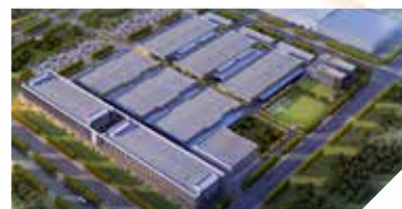
■ 天津工厂(在建中)/Tianjin factory (Under construction) 占地面积/Total land area: 373,000m 2 建筑面积/Total floor area: 300,000m 2
