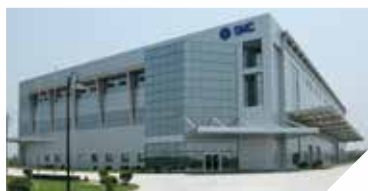
■ 上海工厂/Shanghai factory 占地面积/Total land area: 18,140m 2 建筑面积/Total floor area: 16,173m 2
