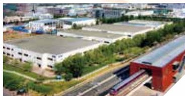
■ 北京第二工厂/The second factory 占地面积/Total land area: 60,589m 2 建筑面积/Total floor area: 40,222m 2
